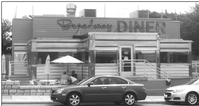
A view of the Broadway Diner in its current location, Baraboo Wisconsin.
